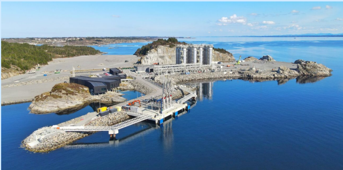
Figure 4: Northern Lights CO 2 import terminal under construction in Øygarden, Norway
