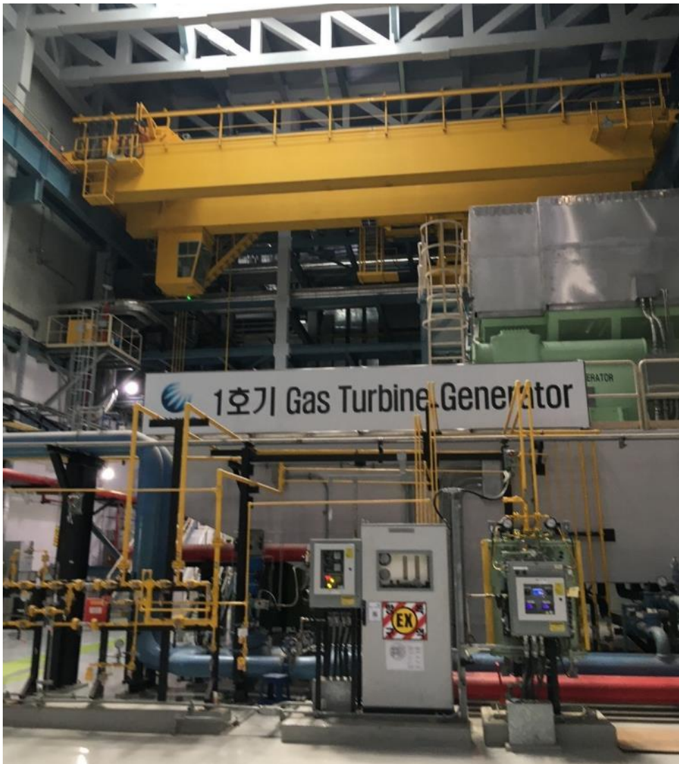
One of two underground gas turbines powering the 800 MW KOMIPO power station in the heart of Seoul.
