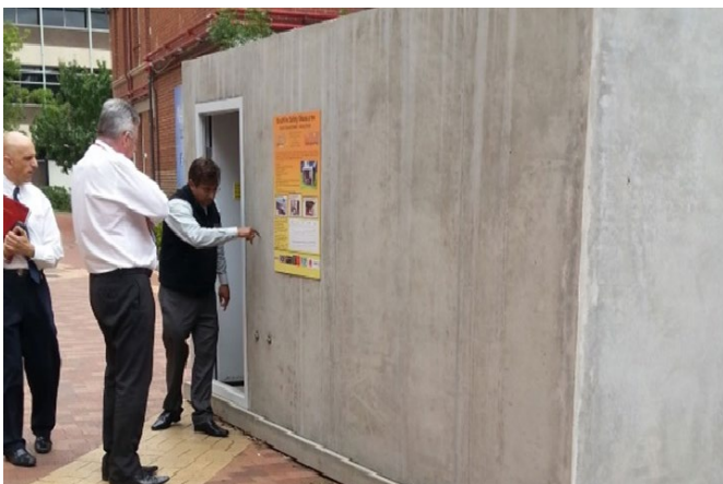
An example of an accredited bushfire bunker before being installed in the ground.
